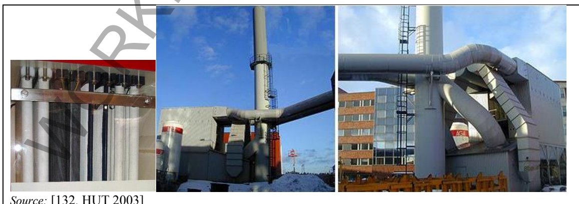
Figure 3.57: Bag filter units; inside (L) and outside (C, R) views
