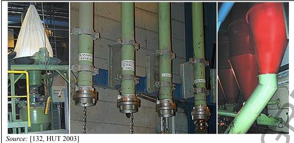
Figure 2.12: Pneumatic conveyors and silos for powdered materials
