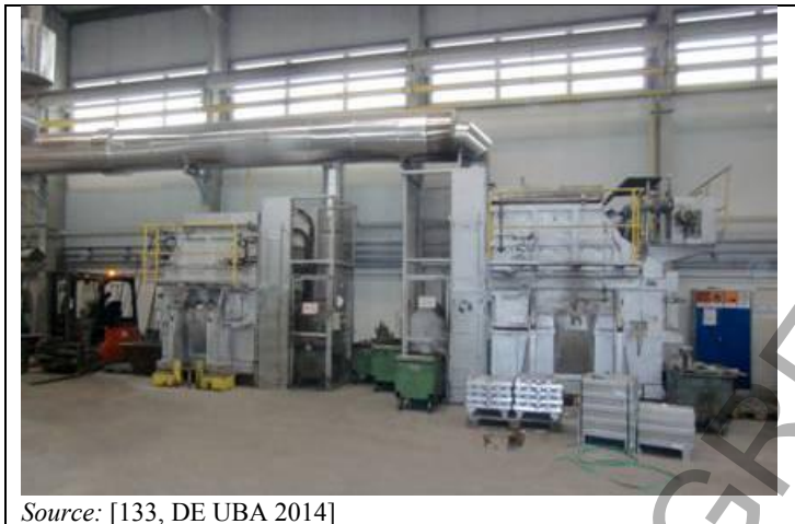
Figure 3.12: Exhaust systems of four furnaces connected with heat exchangers to transmit the heat of the hot gases from the melting process to the heating circuit
